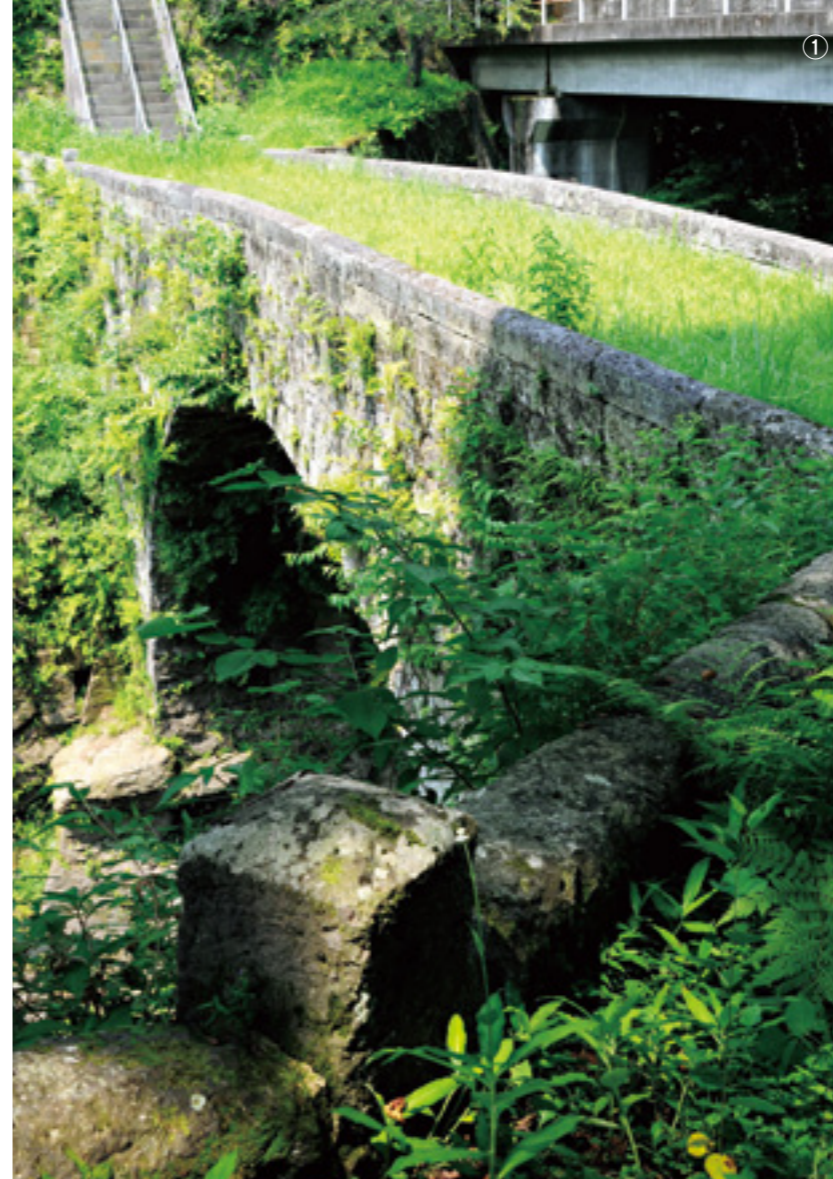
↑ The "Iwato Bridge" built by Kakita Kakujiro, who was a powerful village headman in the Kashiwaru area. (Important Cultural Asset Designated by Oita Prefecture/Completed in the second year of Kaei (1849))
